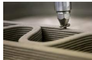
Concrete 3D printing
